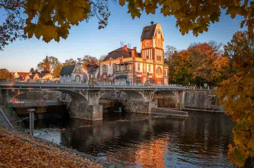
The Elbe Power Station , otherwise known as Hučák , was connected to the power grid on 12 February 1910 at 2 p.m. That same evening, it ceremonially lit the arc lamps in the Great Square.
